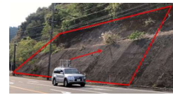
Roadside slope monitoring system
