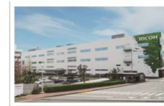
Ricoh Eco Business Development Center in Shizuoka Prefecture
